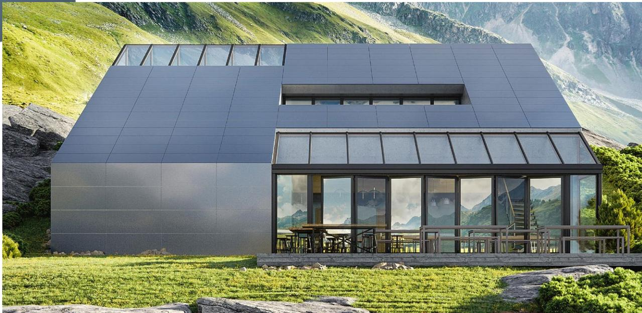
Building integrated photovoltaics in a minimalistic design
